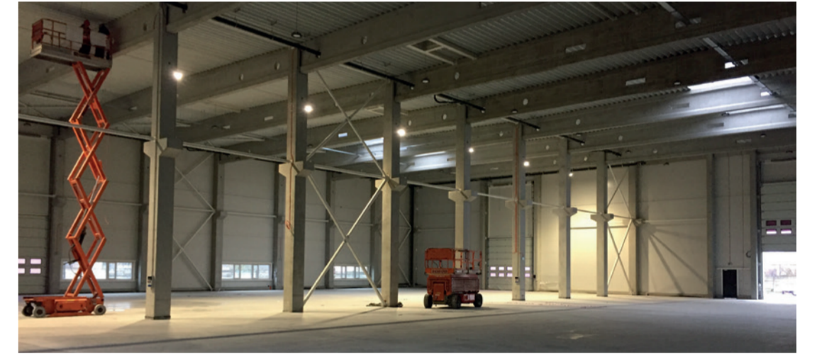
Under construction: MAPLAN plant in Malacky, Slovakia
