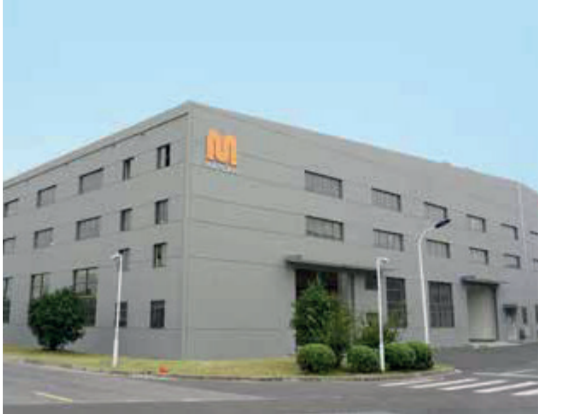
New MAPLAN plant in Wujin, China
